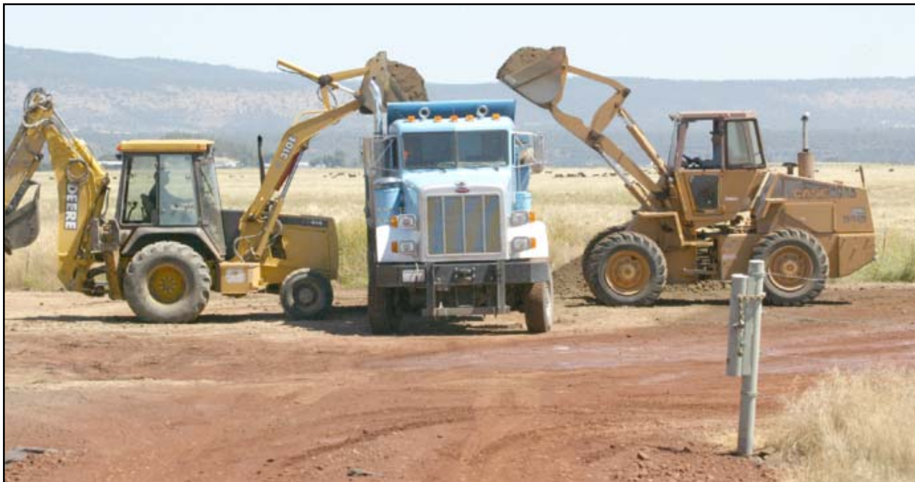
PG&E is moving truckloads of fill out from the existing Rat Farm Road, north of the Inter-Mountain fairgrounds in McArthur, seven days a week during daylight hours. The company said it would take at least three weeks to rebuild the road before they could even get equipment out to the levee that was breached Aug. 3.
