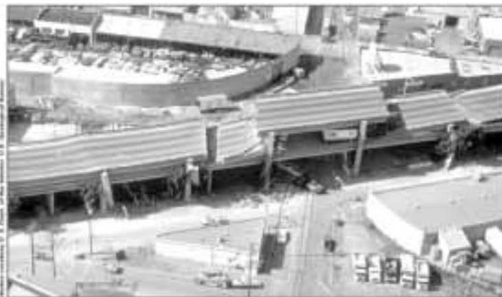
In October 1989, a major earthquake hit in the Santa Cruz Mountains in California, on the San Andreas Fault. It was a magnitude 6.9, and caused 63 deaths and about $6 billion in damage. ("Magnitude" is a measure of how powerful an earthquake is.) This freeway was torn apart by the quake.
