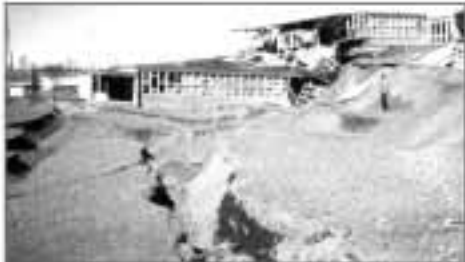
The largest earthquake to hit in the U.S. was in the waters off the coast of Alaska in 1964. It was a 9.2 magnitude and caused much damage in Anchorage, including this elementary school, which was destroyed by a landslide during the quake.
